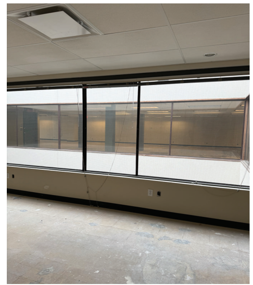
2nd & 3rd Floor Skylight Well
